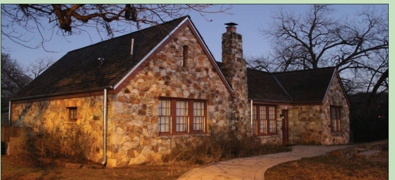
PARK'S HOME Zilker Caretaker's Cottage remains one of the oldest standing structures from the beautification that occurred in the '30s. The cottage now serves as Park Rangers headquarters. photo by JC Ramirez Delgadillo
