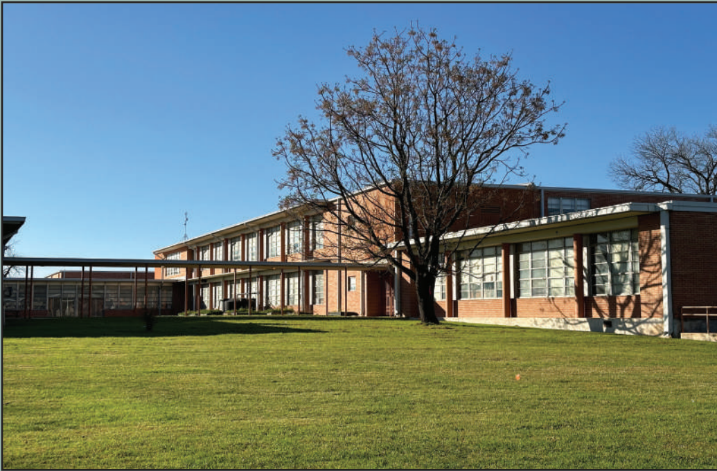
EXPENSES SOAR The Anita Ferrales Coy Facility, currently hosting AISD’s Alternative Learning Center, will be torn down to create housing opportunities for AISD teachers and staff. The renovated facility will be home to two new apartment complexes with a total of 500 housing units and a renovated ALC. photo by Lily Wilkerson
