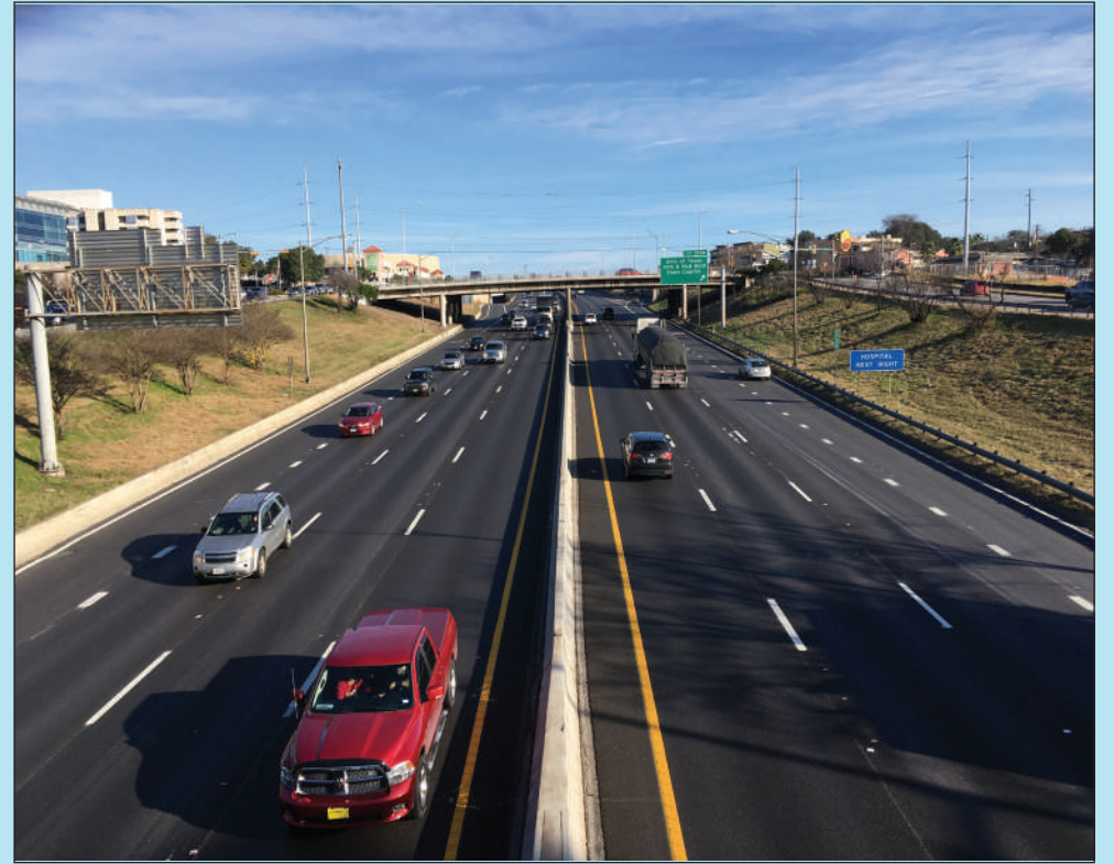
DRIVING AROUND Interstate-35 plays a major role in many Austinites' daily commutes, connecting San Antonio to Austin. A decade-long renovation plan has been approved by the city of Austin to expand the highway, adding 10 lanes, in some stretches of the road. photo by Lily Wilkerson
